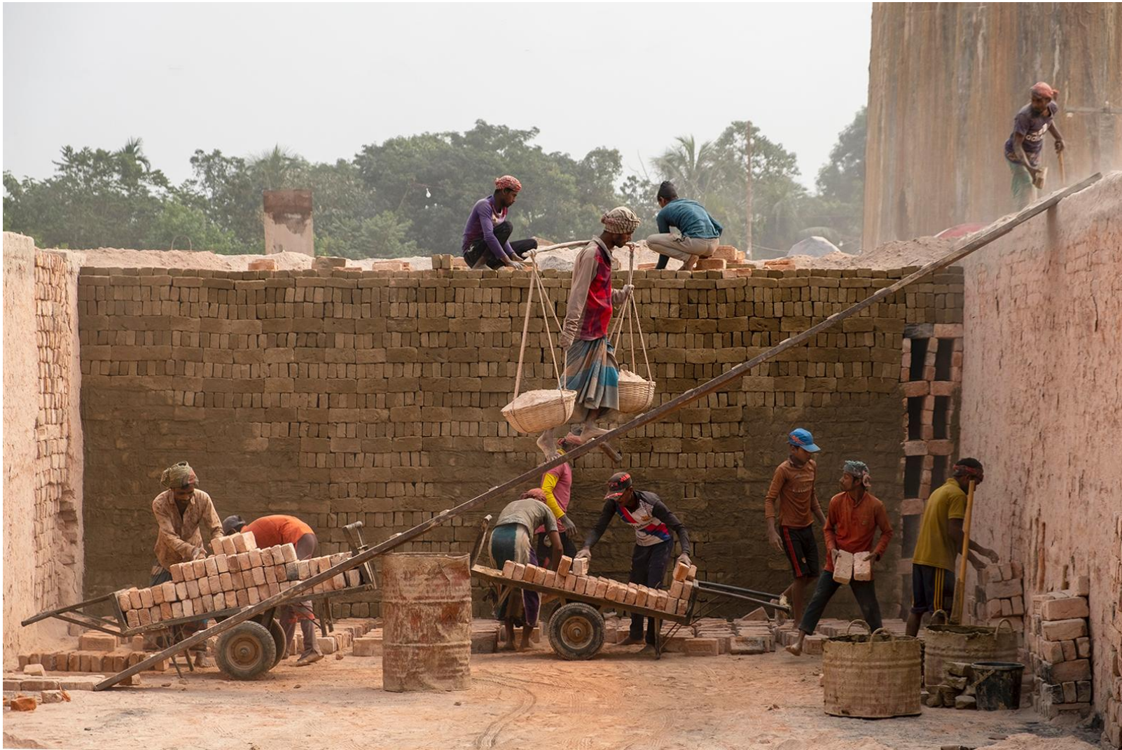
NPS e-HM | BUSINESS AT BRICKFIELD | MD. IQBAL HOSSAIN | Bangladesh
